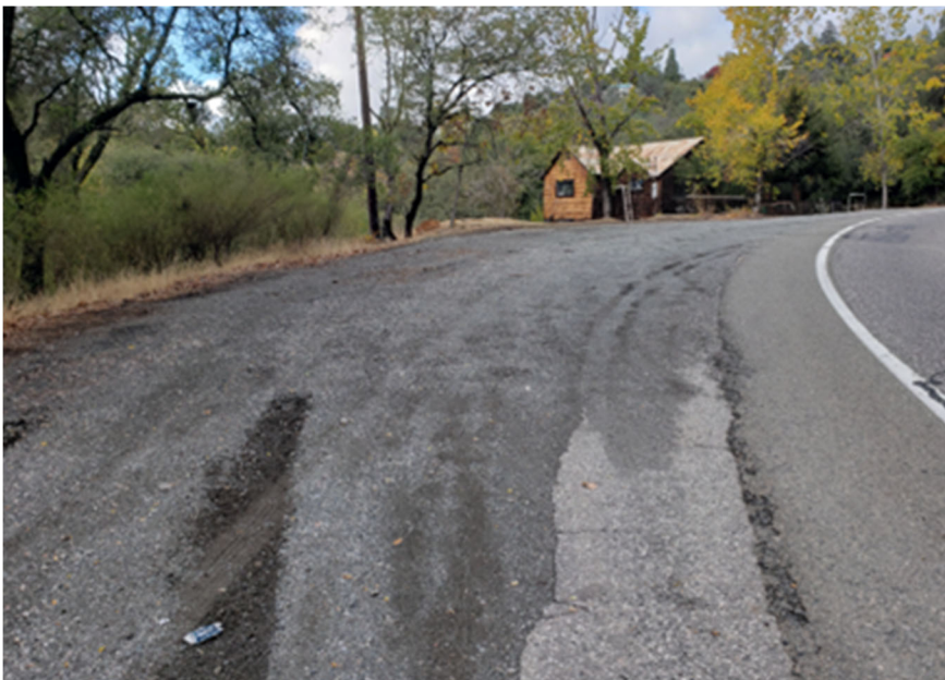
FIGURE 38: PHOTO OF SR 49 NEAR PM 2.0 EASTBOUND
