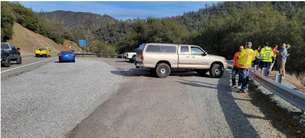
FIGURE 44: PHOTO OF SR 49 NEAR PM 0.7 EASTBOUND
