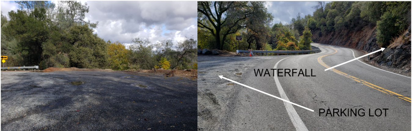
FIGURE 43: PHOTO OF SR 49 AT CANYON CREEK EASTBOUND
