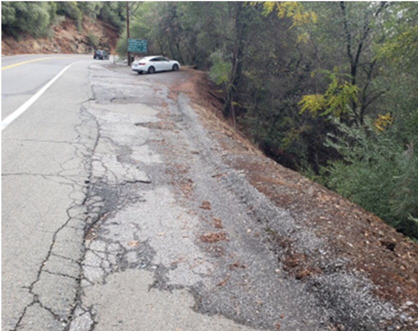
FIGURE 37: PHOTO OF SR 49 PULLOUT AREA NEAR PM 2.15 HEADING EASTBOUND
