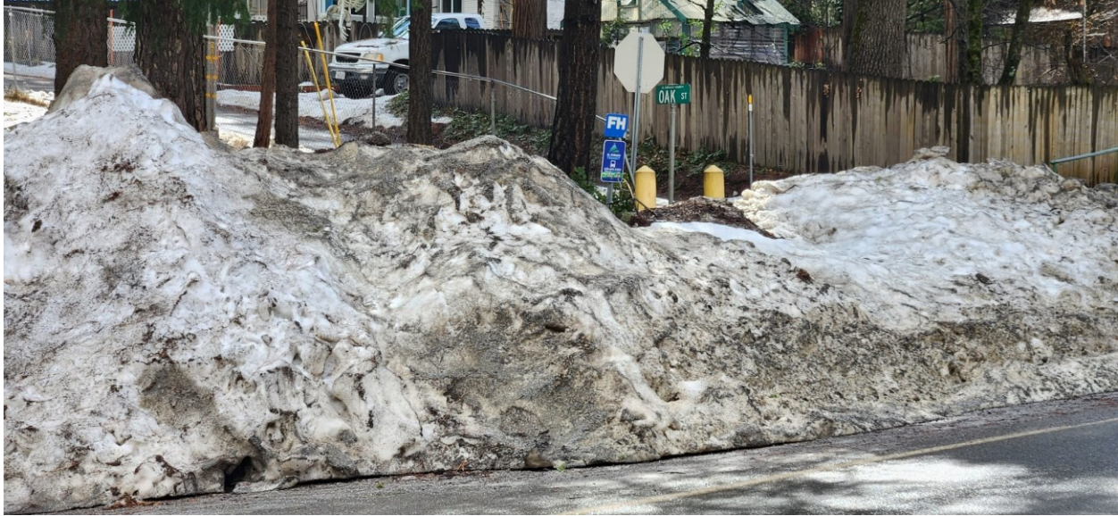
Figure 14 - Example of Bus Stop without Safe Waiting Area and with Sign Partially Obscured by Plowed Snow
