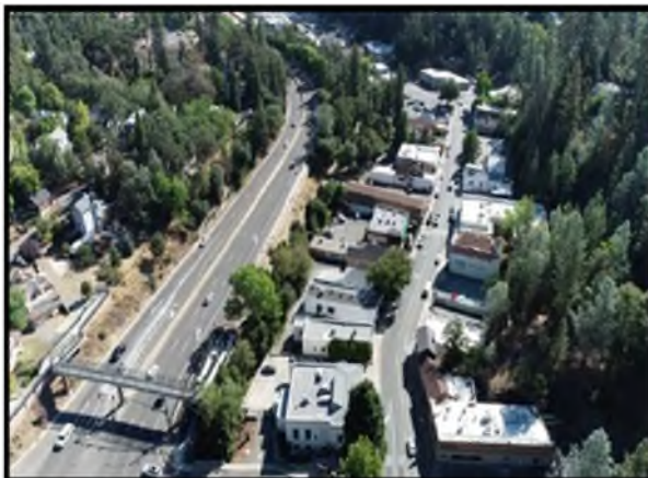
Drone image showing free flowing traffic on US 50 during Trip to Green Operations on October 1, 2022
